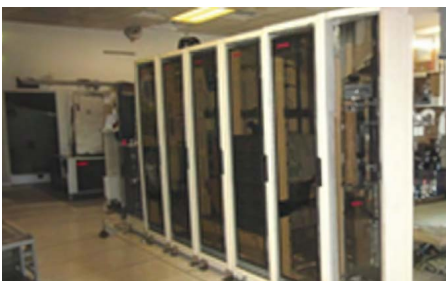
Computer server racks anchored to the floor.
