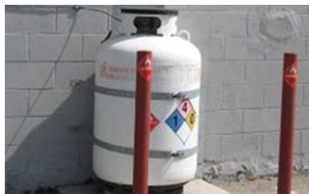
Flammable liquid tank strapped to wall.
