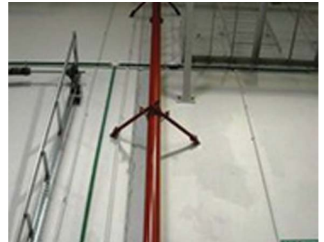
Sprinkler riser with sway bracing.
