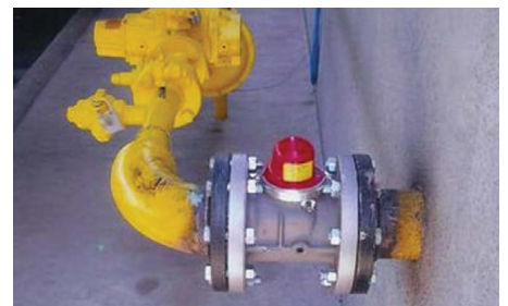
Seismic shutoff valve for natural gas line.
